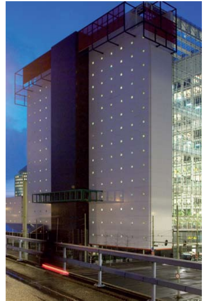
Ministry of Infrastructure and the Environment Rijnstraat 8
